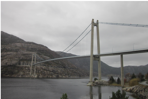
Figure 1: South view of the Lysefjord Bridge.
